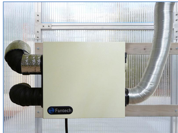
Heat recovery ventilator
