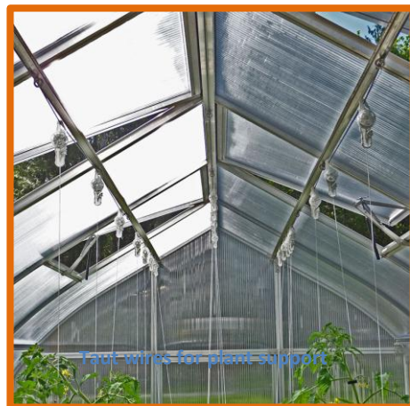
Three overhead taut wires
