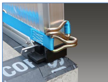
Hold gable edges in place
