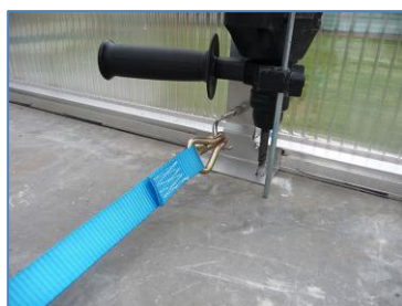
Restrain mounting brackets
