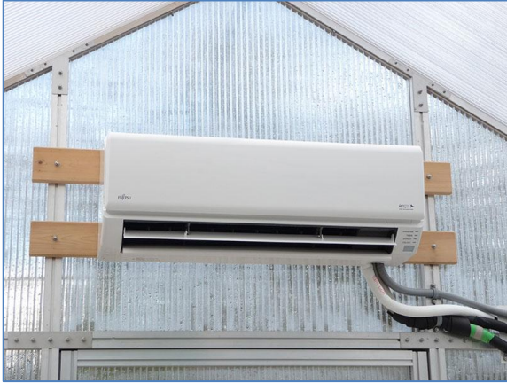
Ductless mini-split heat pump indoor unit
